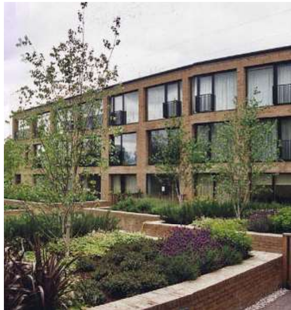
Brick built blocks with large windows
