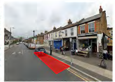
Location of parklet structure highlighted in red
