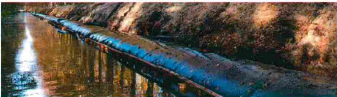
Dredged silts stored in the silt bags at a greater depth and density than when loose in the water body.
