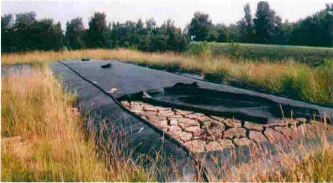
Dried silts being cut from the silt bags to be used in landscaping.
