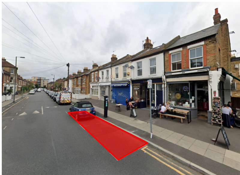
Location of parklet structure highlighted in red
