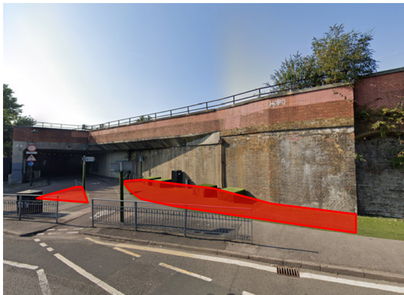
Location of parklet structure highlighted in red
