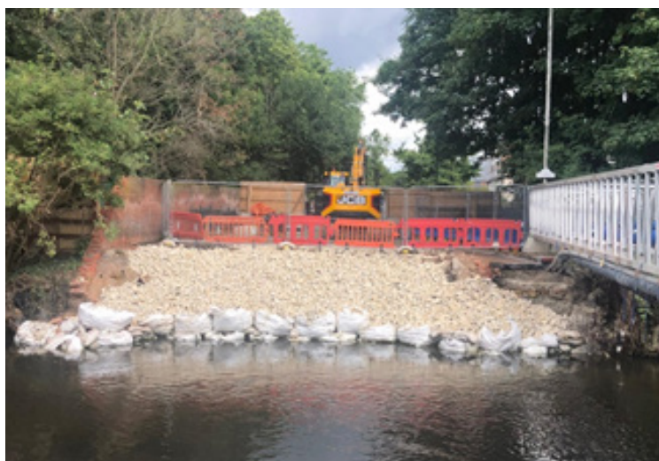
Photo of demolished bridge with gantry for utilities to the right
