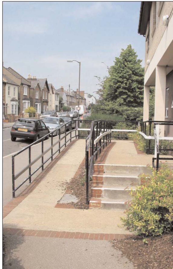
(Below) 42-44 Russell Road, Wimbledon.
