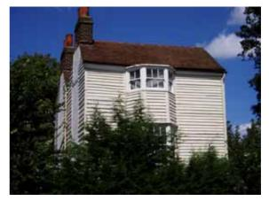
Part brick/part timber construction typical of a number of buildings in the area including timber-framed buildings, possibly originally weather boarded, with either an external brick skin or render on lathes to give the impression of a more solid construction, of which nos 4-8 Merton High Street are examples.
