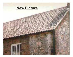
parallel with the front of the building, for example White Cottage in Morden Road. Roof coverings include a few examples of red pantiles mainly to timber framed buildings. Plain clay tiles and Welsh slate, however, became increasingly widespread from the later part of the 18th Century on wards. Flashings are predominantly of lead.
